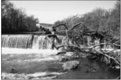
This low-head mill dam on west Conowago Creek in York County was slated for removal in late 2002.
